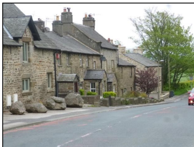
Photo 6. Stone Cottage, Main Road, Slyne
