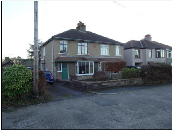
Photo 13. Semi-detached Houses on Kirklands
