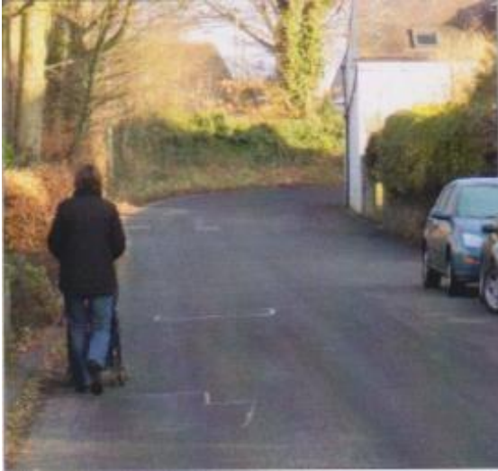
Photo 36. No pavements on Hatlex Lane
